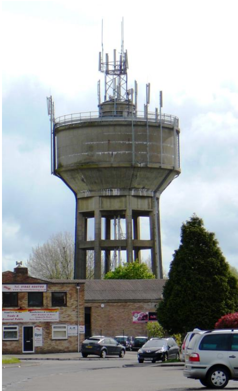
The village water tower with communications antennae.
